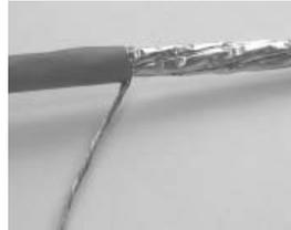
4c. Remove foil from pairs of cable. Twist braid and wrap around the cable sheath
