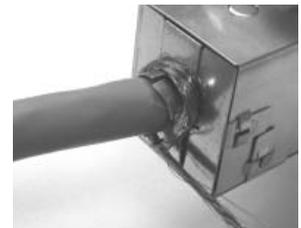
5c. Secure the cable and braid with the plastic cable clamp, place and tighten over the metal cable collar.
