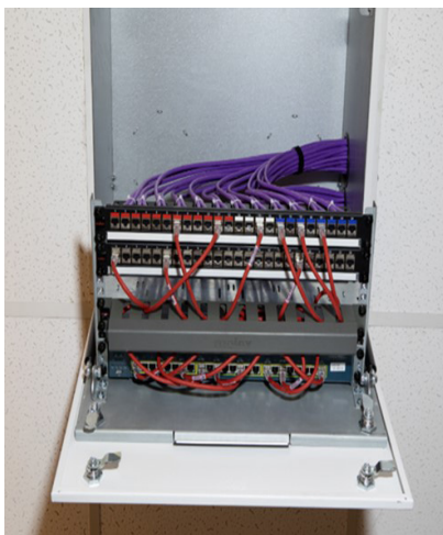
Active equipment installation
