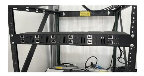
**Step 5.** Ground the MultiGate by connecting a wire between the grouding screw and chassis of the rack.
